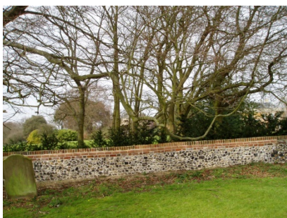
Repaired Churchyard West Wall
