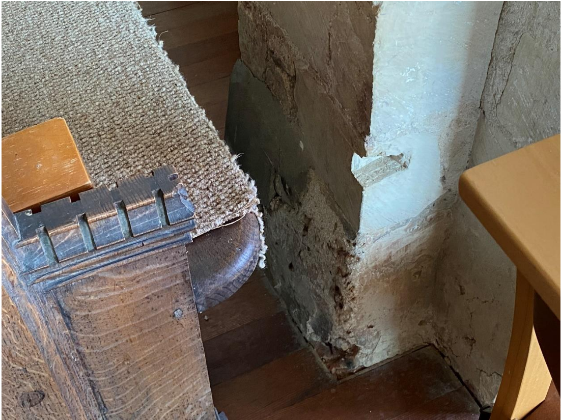
11.10 Nave south pier
