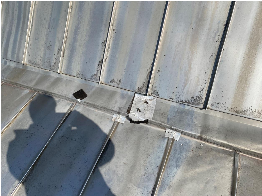
7.12 South aisle roof
