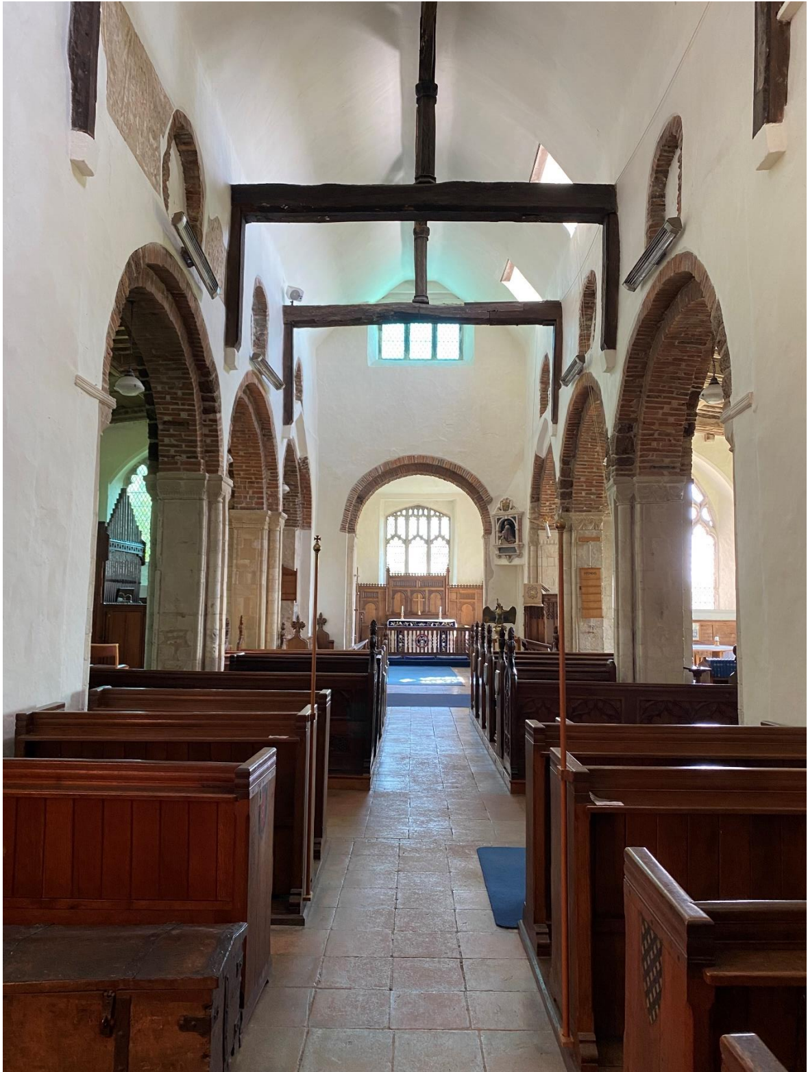
Interior looking east
