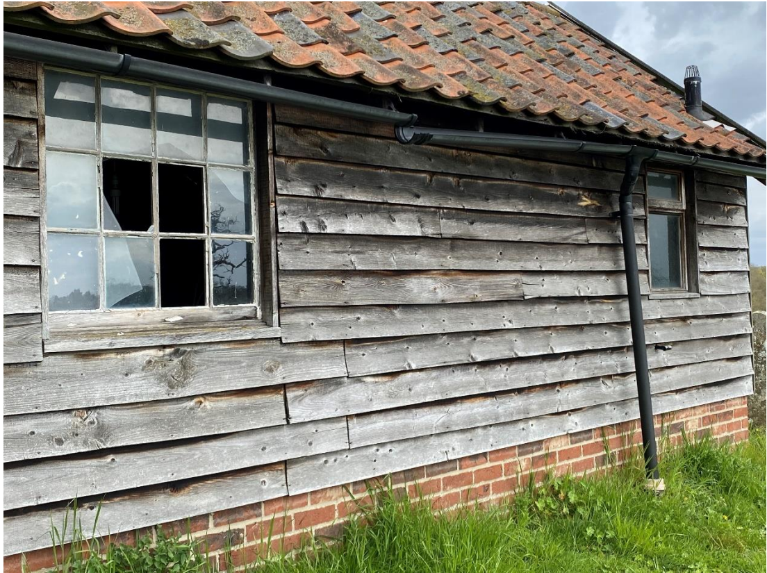
15.18, 15.9 Outbuilding gutter and window
