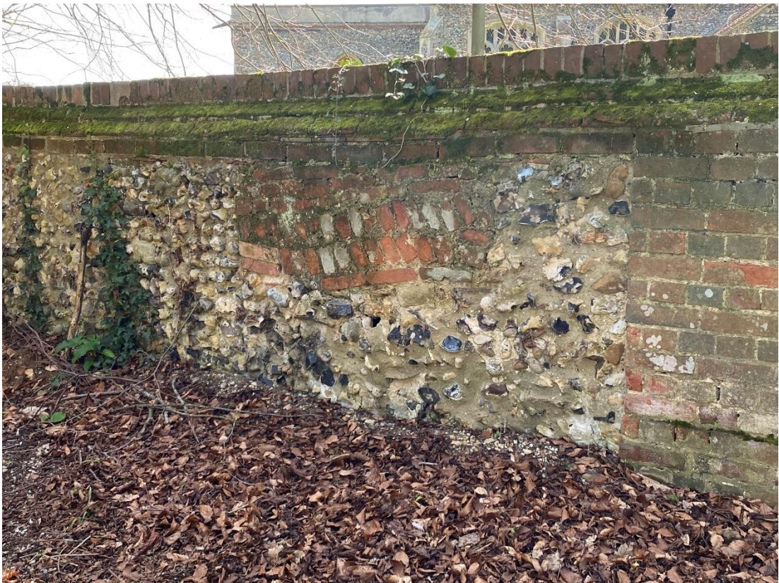
15.6 North boundary wall north face
