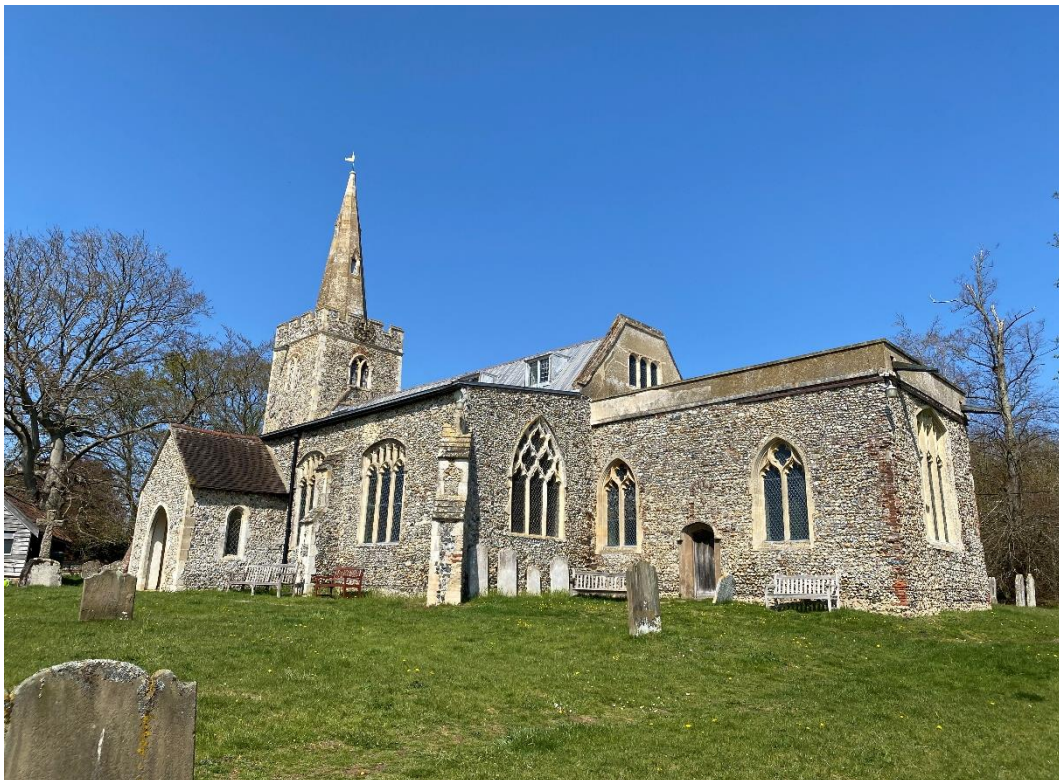
Exterior from south east
