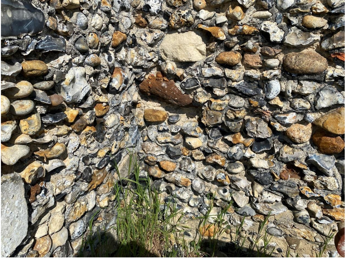
8.19 South aisle south elevation (typical)
