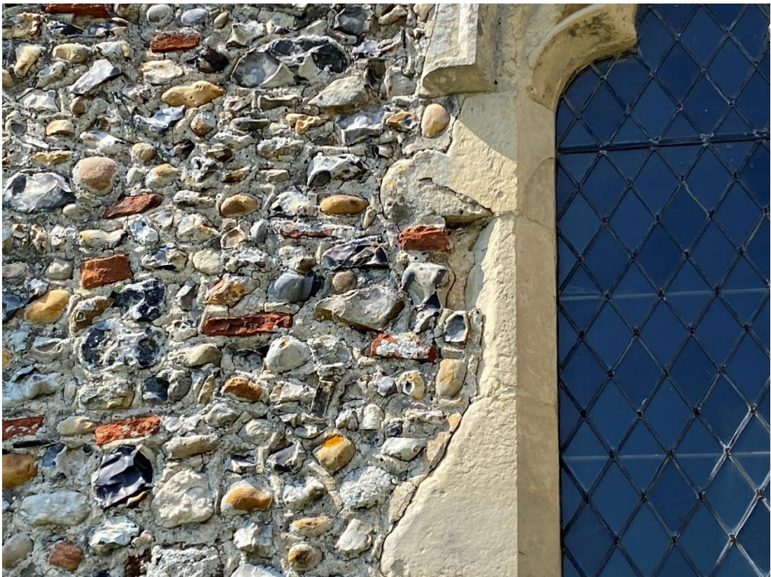
8.18 South aisle east elevation
