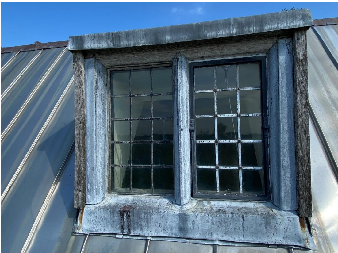
9.12 Nave south window (east)
