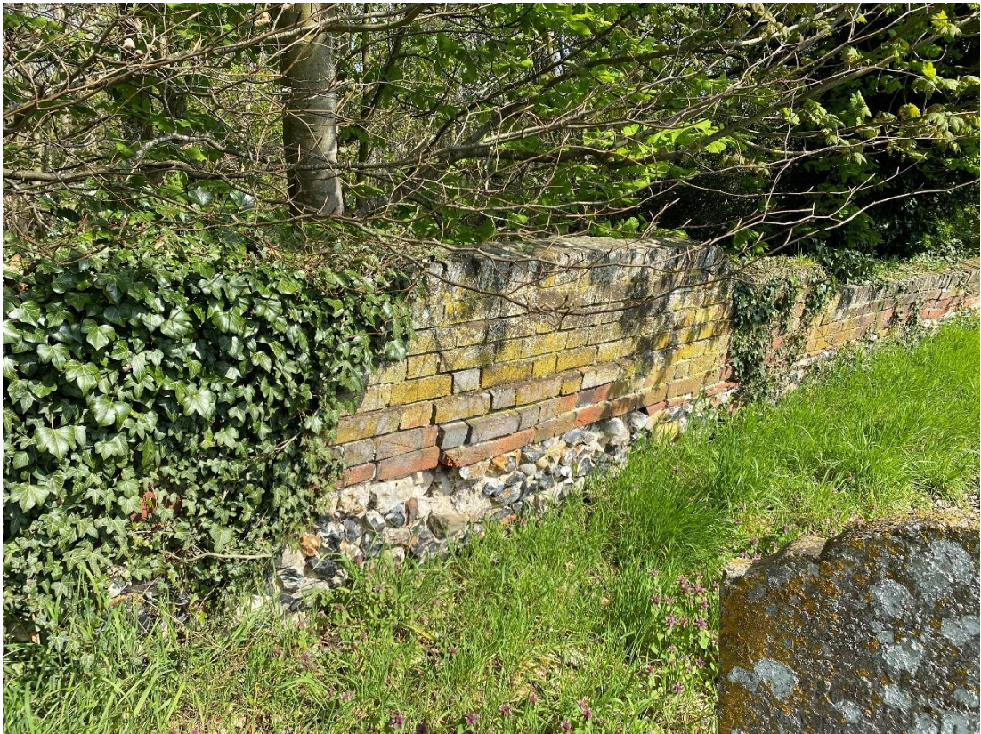
15.8, 15.9 North boundary wall east section
