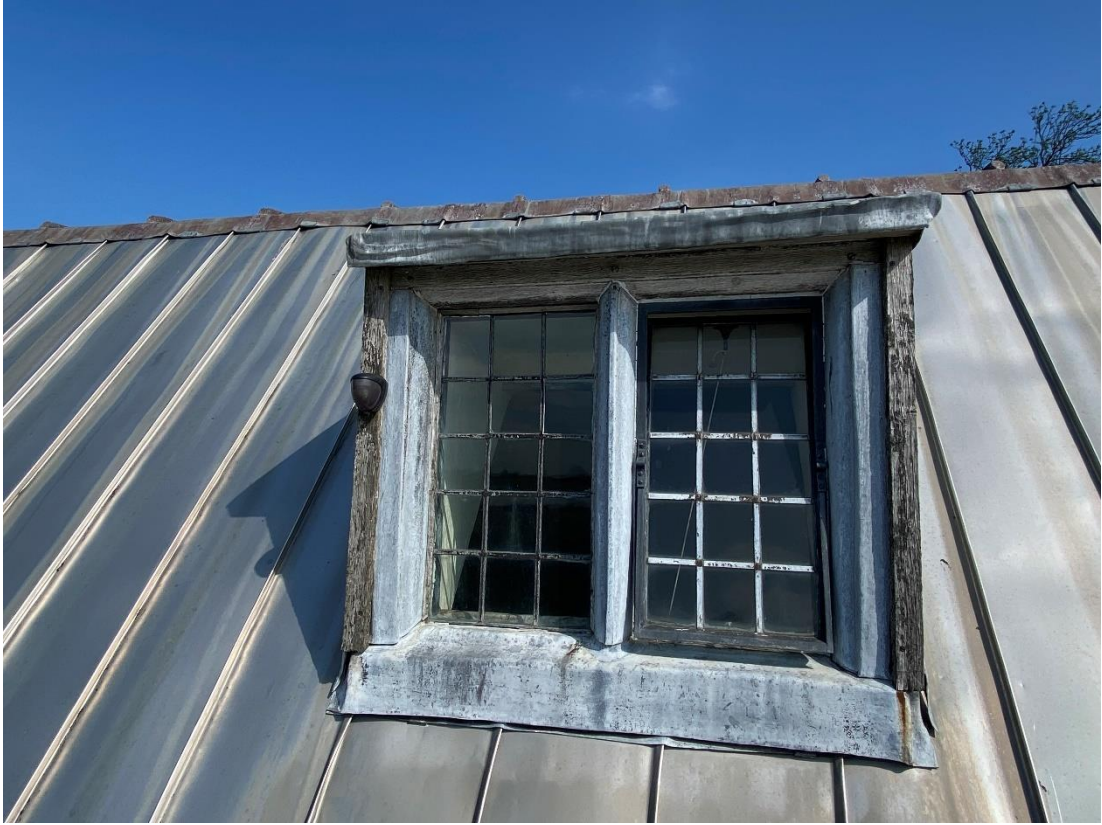
9.12 Nave south window (centre)
