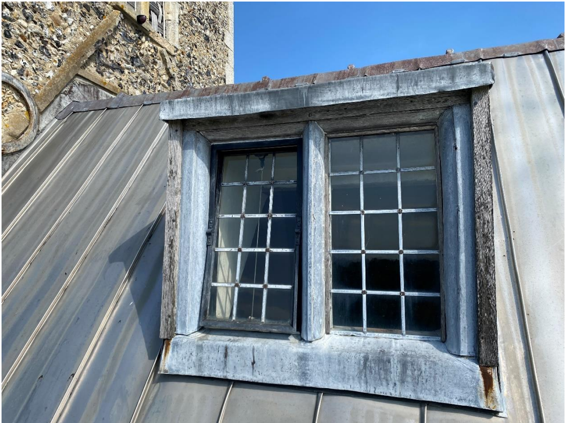
9.12 Nave south window (west)
